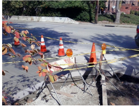
Figure 8.1: A wooden spline used to create a smooth, curved border for a paved area (Shadyside, Pittsburgh, October 2014).
