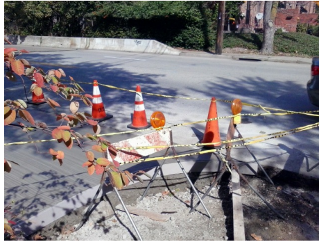
FIGURE 8.1: A wooden spline used to create a smooth, curved border for a paved area (Shadyside, Pittsburgh, October 2014).
